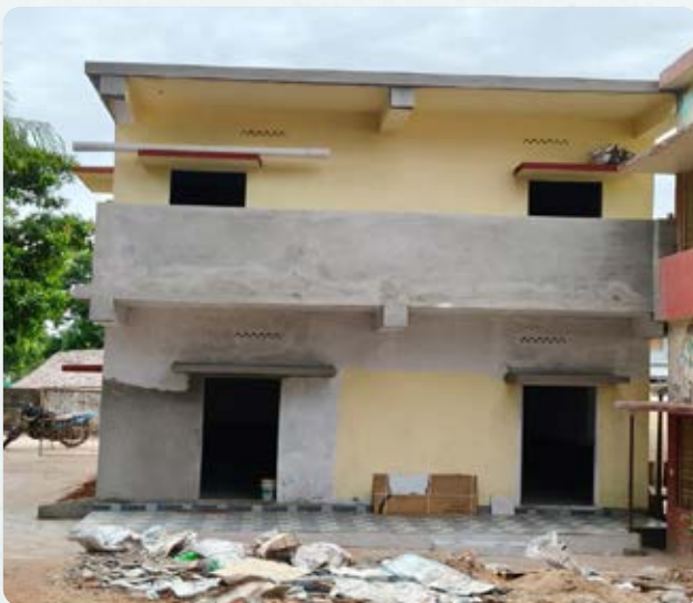
Construction of new classrooms for City Municipal Corporation High School, Morumpudi.
