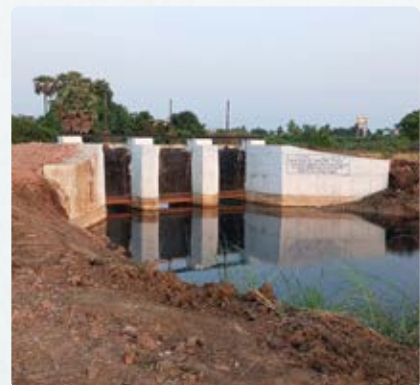
Constructed small dam to block excess waterlogging in paddy fields during rainy season
