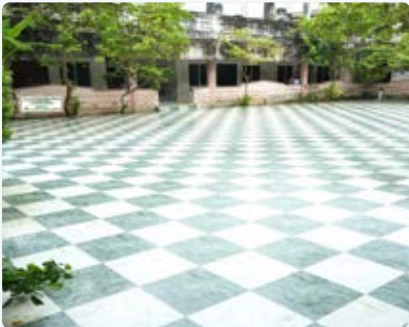
Inside hostel flooring
