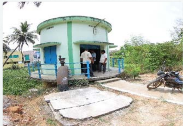
Constructed sump cum pump house and main water line at kotilingalapeta, RJY to prevent flooding in rainy season.
