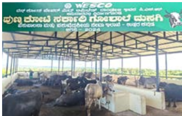
Construction of Goushala at Dusagi Village
