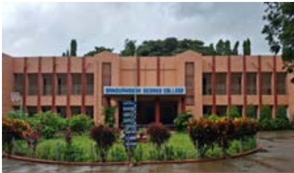
Renovation of Bangur Nagar Degree College at Dandeli
